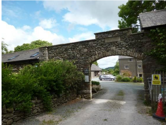
Fig.19: 1914 archway from south with Firbank Fell to left
