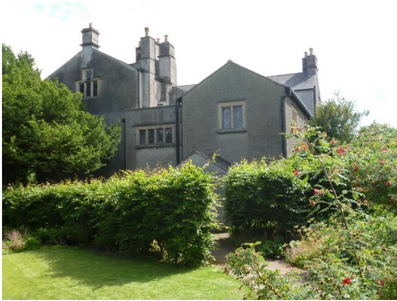
Fig.9: north elevation with 1914 extension to right, 2016
