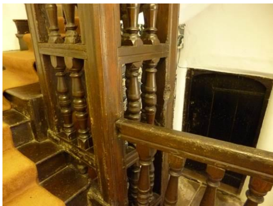
Fig.10: caged newel staircase
